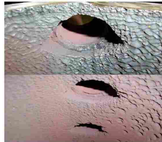
Figure 3-2 Example of Severe Ongoing FAC Damage (Above) – Black Magnetite Covered Surfaces, Example of Previous FAC Damage Now Protected (Below) – Red Hematite Covered Surfaces
